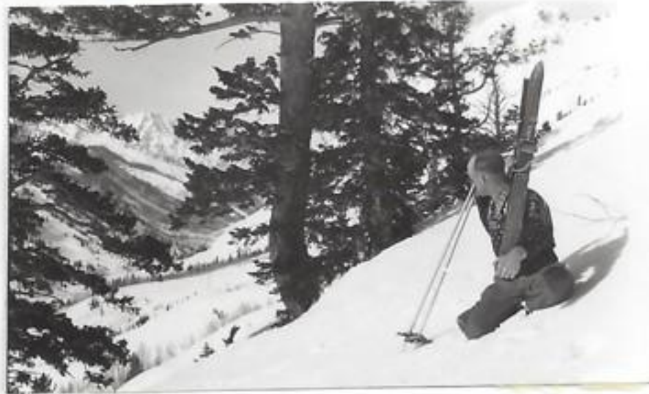
PHOTO 2-2-23-46 James W. Bee near top N ridge. These trees on slope provide relatively safe ascent.
