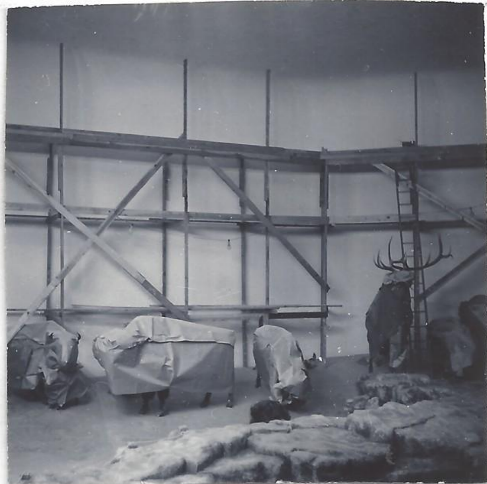
551127-10 Grassland before sod was placed on floor
