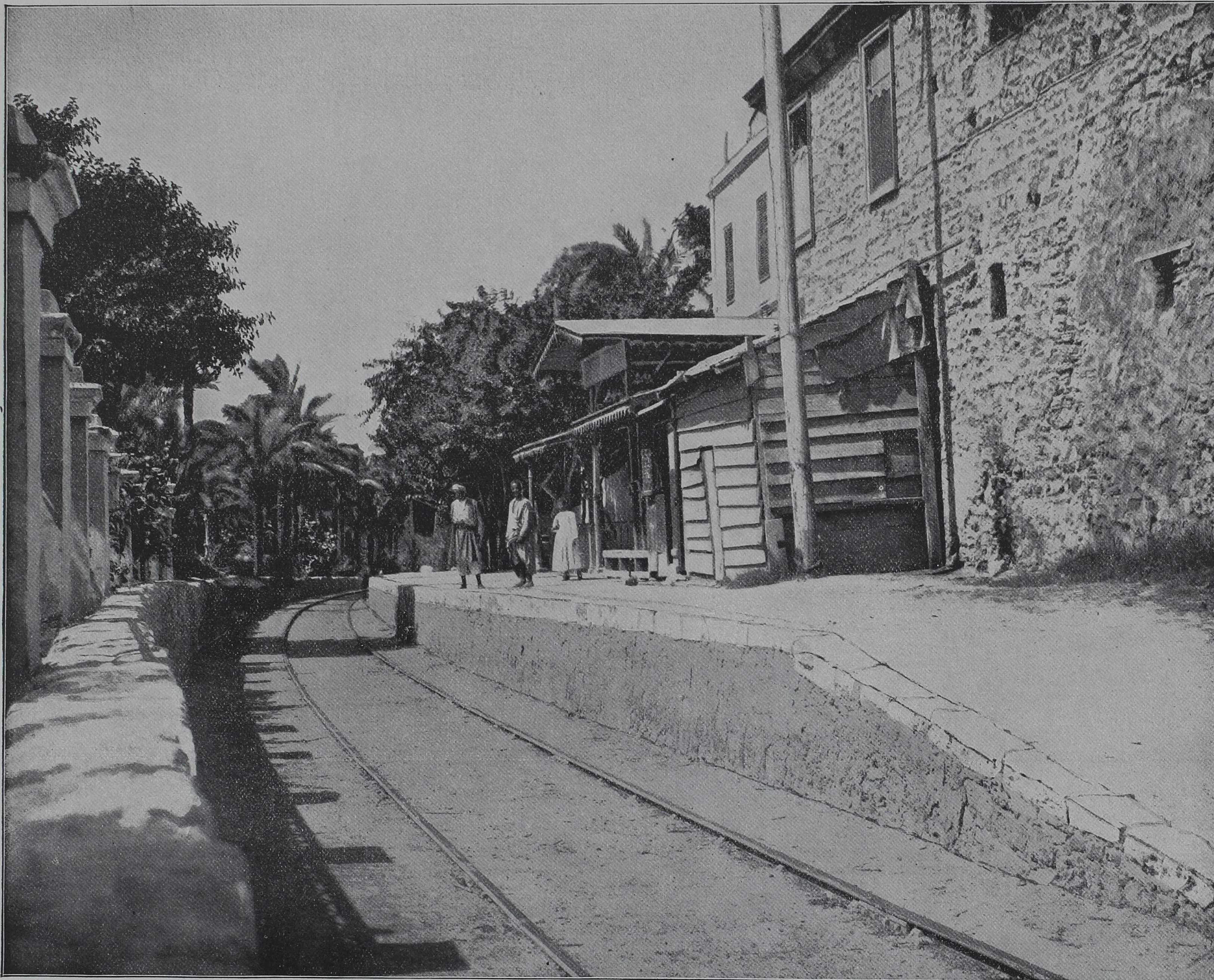
STATION, RAMLEH, PALESTINE. —On the direct route from Jaffa to Jerusalem is the town of Ramleh, which is said to occupy the site of the ancient Arimathea. Under the Arabs in the ninth and tenth centuries it was a prosperous and important place, and was larger than Jerusalem itself. To-day it contains about 3,000 inhabitants, of whom 1,000 are Christians of the Greek Church. There is an old Latin monastery here, where travelers are lodged and fed with comparative comfort. A lofty tower also rises above the town and once formed part of an enormous Mosque. The country around Ramleh is remarkably fertile. The vegetation is luxuriant. Olive trees abound, and with proper cultivation the fields in this part of Palestine could produce crops of which any country might be proud. The most astounding innovation here in recent times has been the railroad , which has already advanced beyond Ramleh and will eventually connect Jaffa with Jerusalem, thirty-three miles away! Within a short time, therefore, the old methods of horse-back riding and carriages over this part of the Holy Land will be discarded. A locomotive will transport tourists across the plain of Sharon; a railroad bridge will span the brook where David chose the smooth stones for his conflict with Goliath; and the conductor may call out to passengers, "Ramleh, residence of Joseph of Arimathea. Five minutes for refreshments!" On the ground of sentiment, however, most people will regret to have a locomotive's whistle wake the echoes of Mount Zion. Here it is the old which interests us, not the new; and steam-cars seem unsuited to the land of Abraham.
