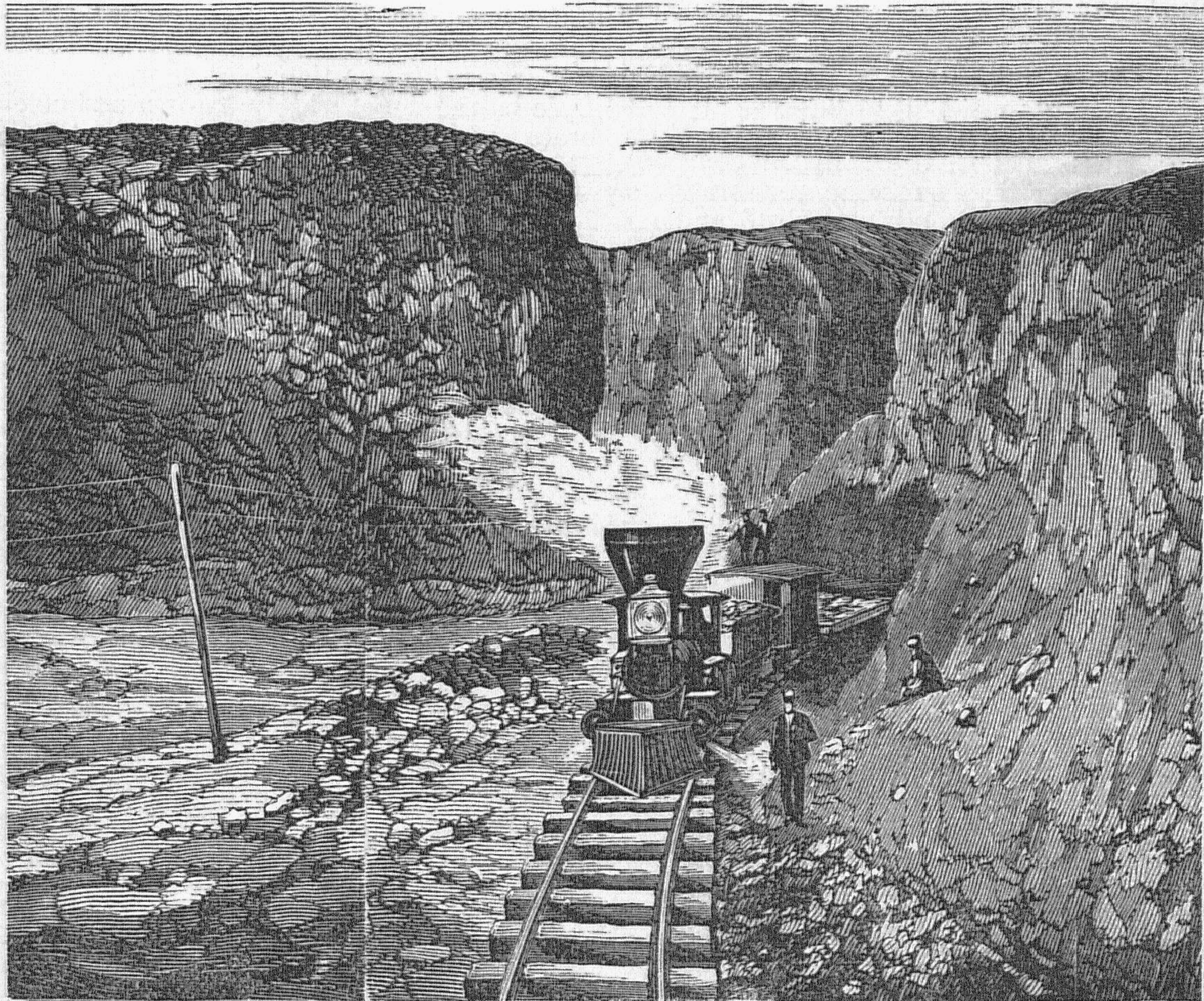
PALISADES OF THE HUMBOLDT RIVER, C. P. R.R.
