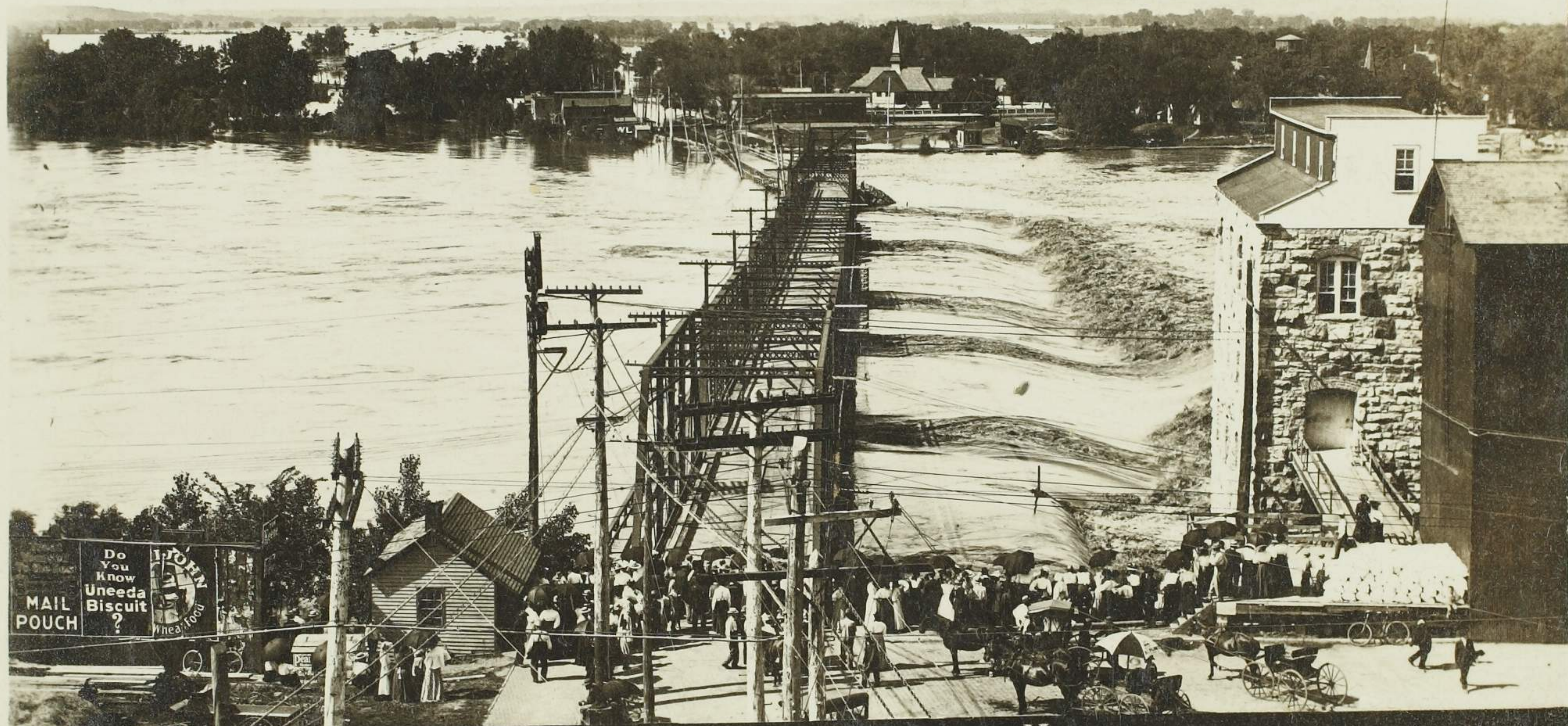
202 Looking North Over Dam, '08 Flood—Lawrence, Ks
