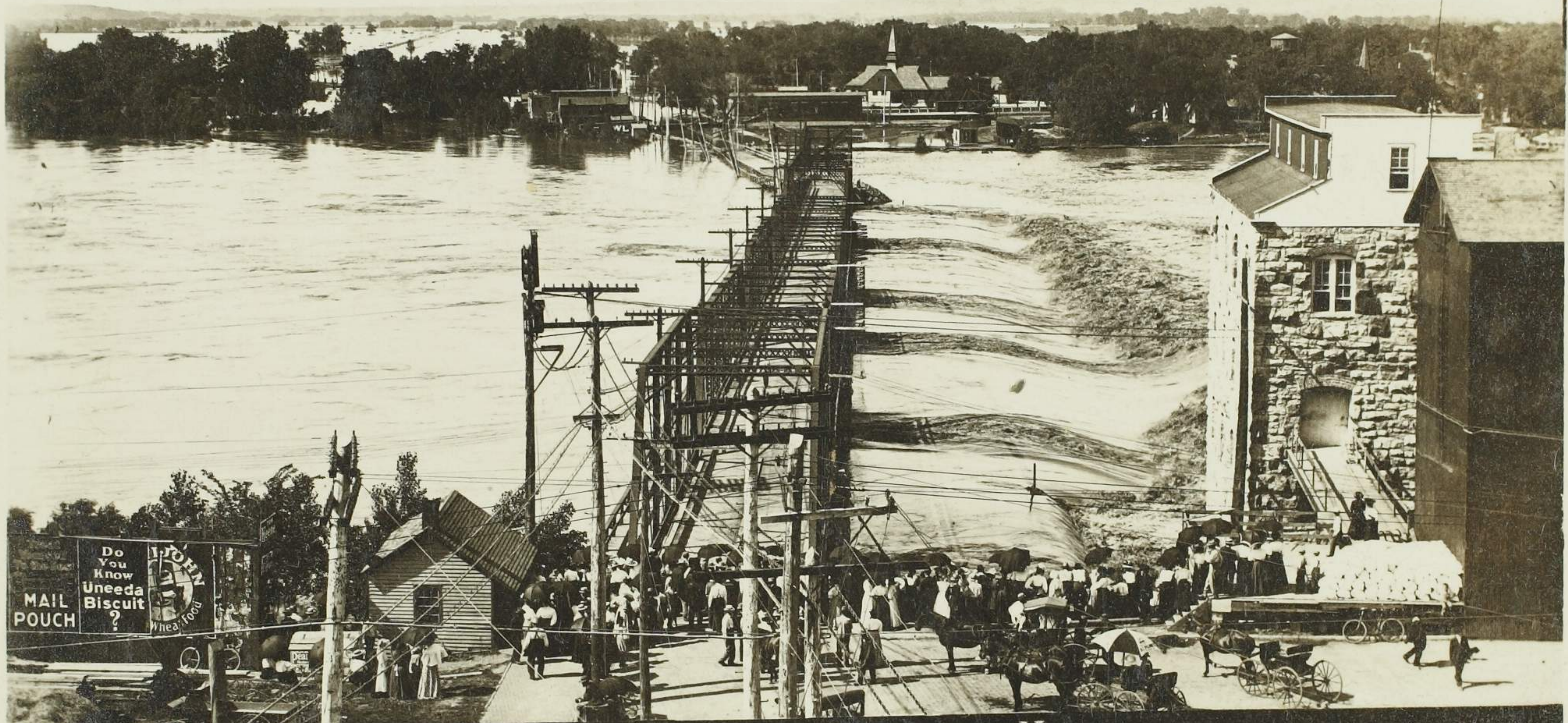
202 Looking North Over Dam, '08 Flood—Lawrence, Ks
