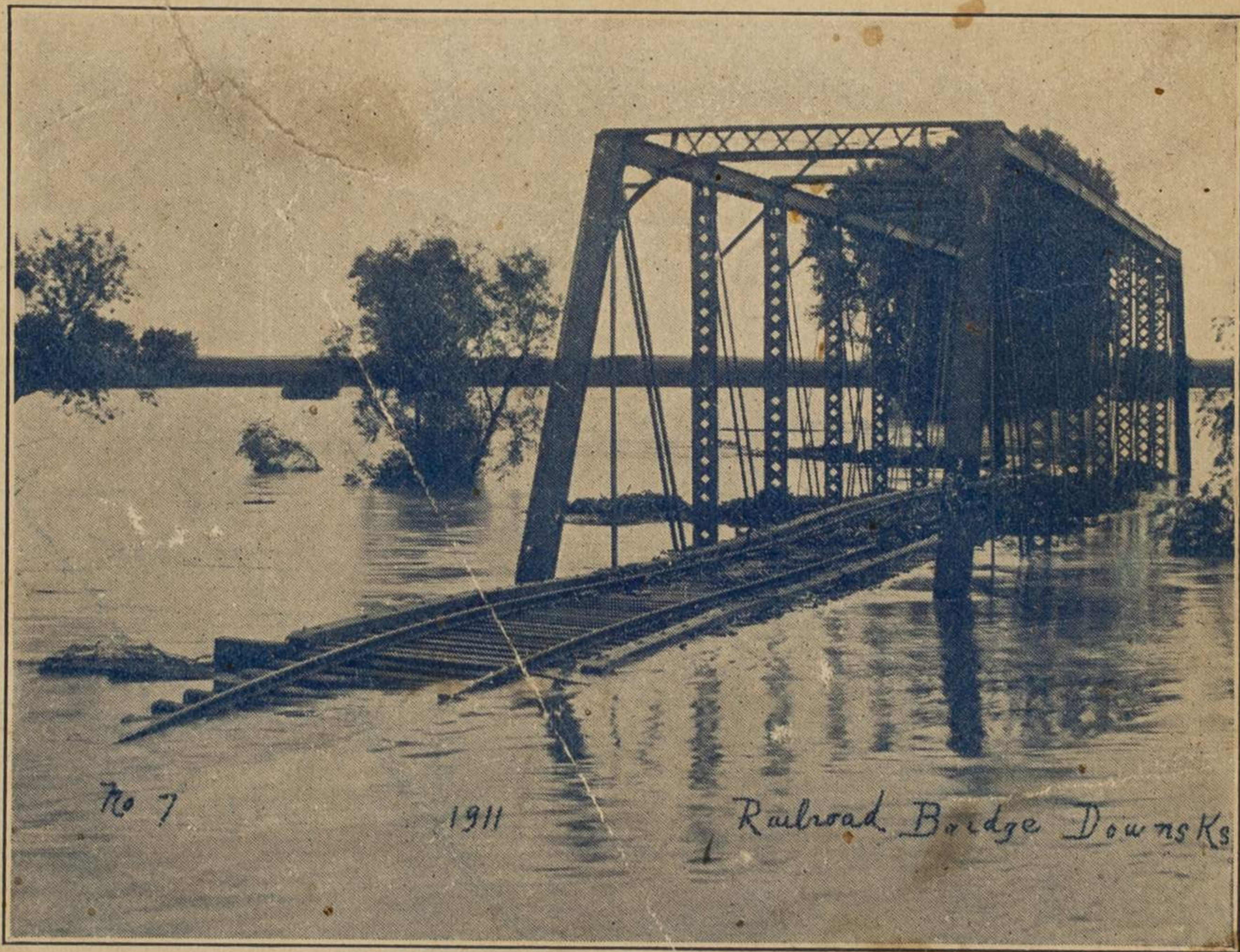
Railroad bridge at Downs, Kansas, on Central Branch, over Solomon river, during flood of August 3, 1911—one-fourth of a mile of grade washed out
