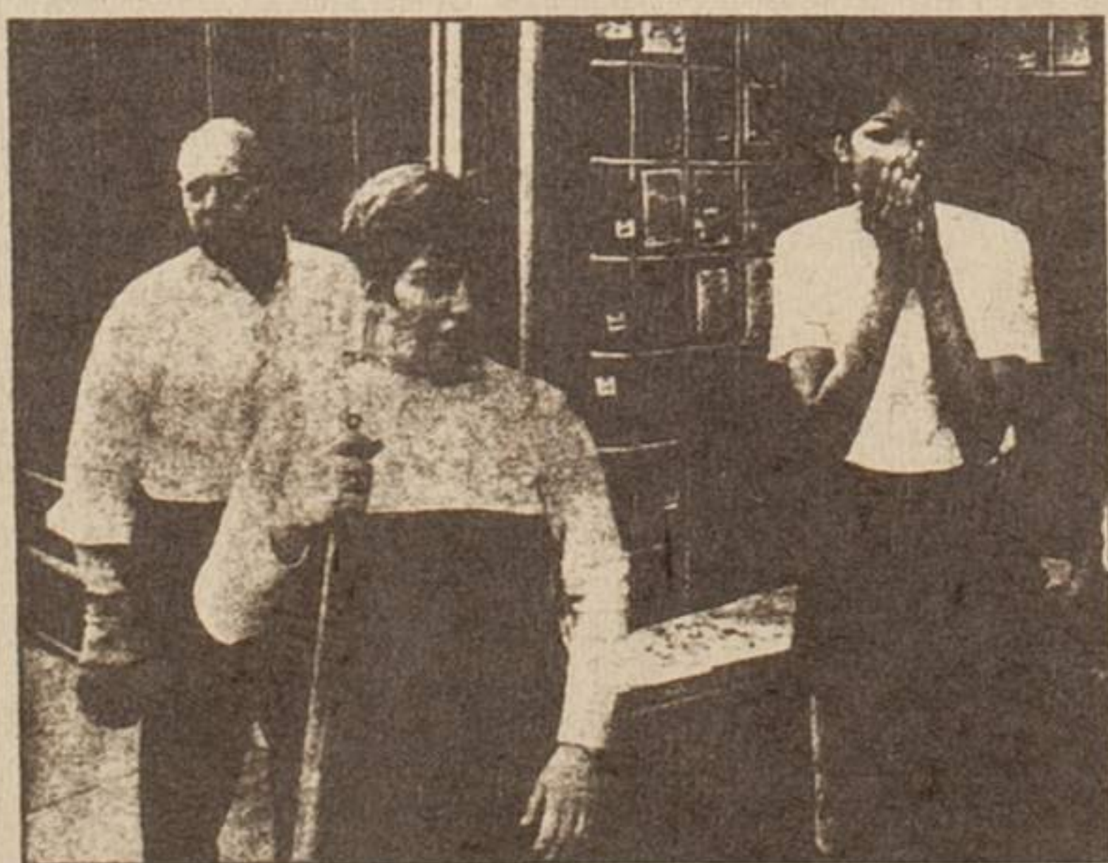
Abe Schwab (left), Beverly Schwab and Michelle Johnson react in astonishment at the sight of armored military vehicles on Beale Street on March 29, 1968. They were cleaning up glass from windows broken the day before at Schwab Brothers at 163 Beale.
