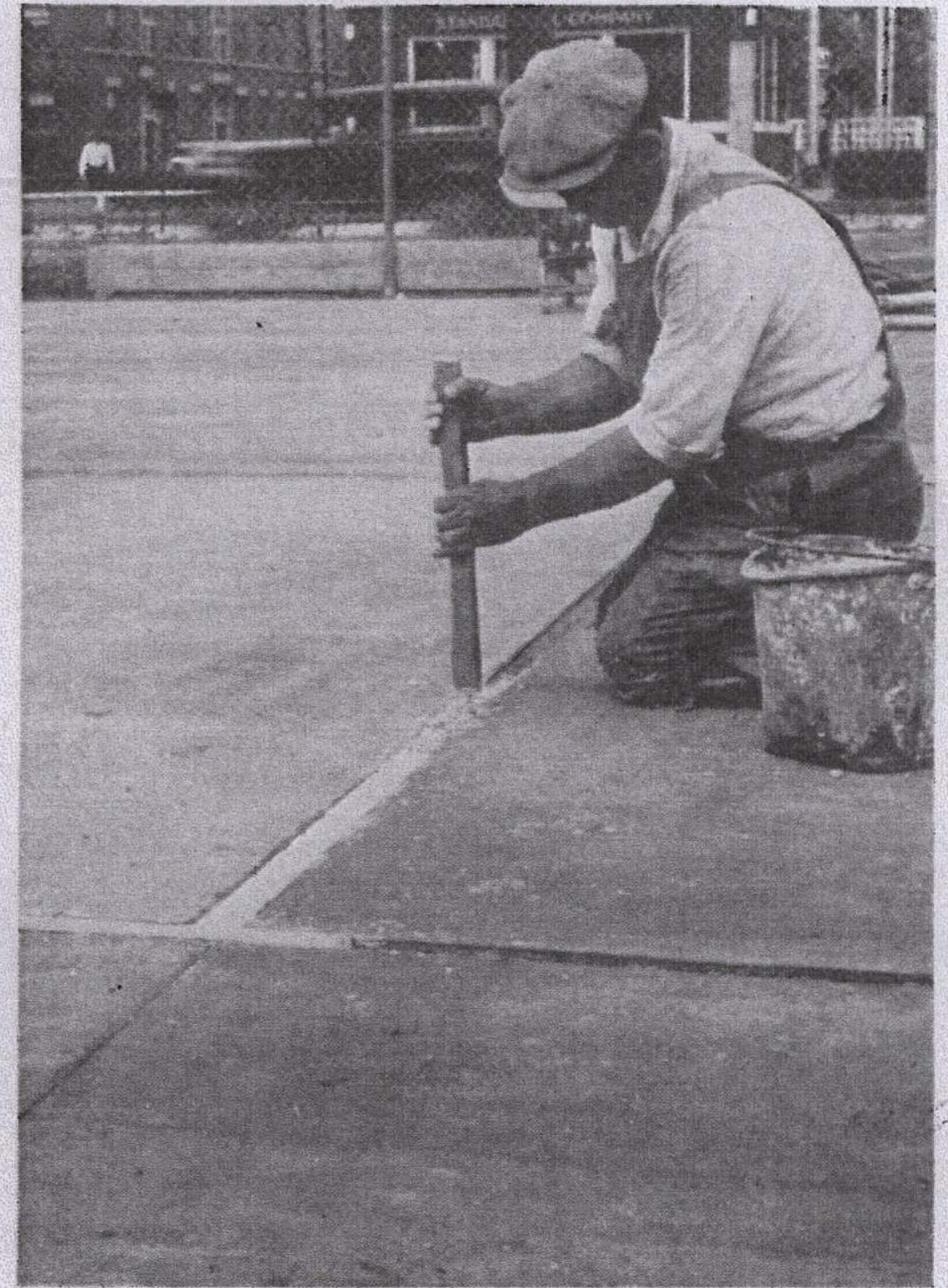
Tamping white portland cement mortar into grooves at lines.
