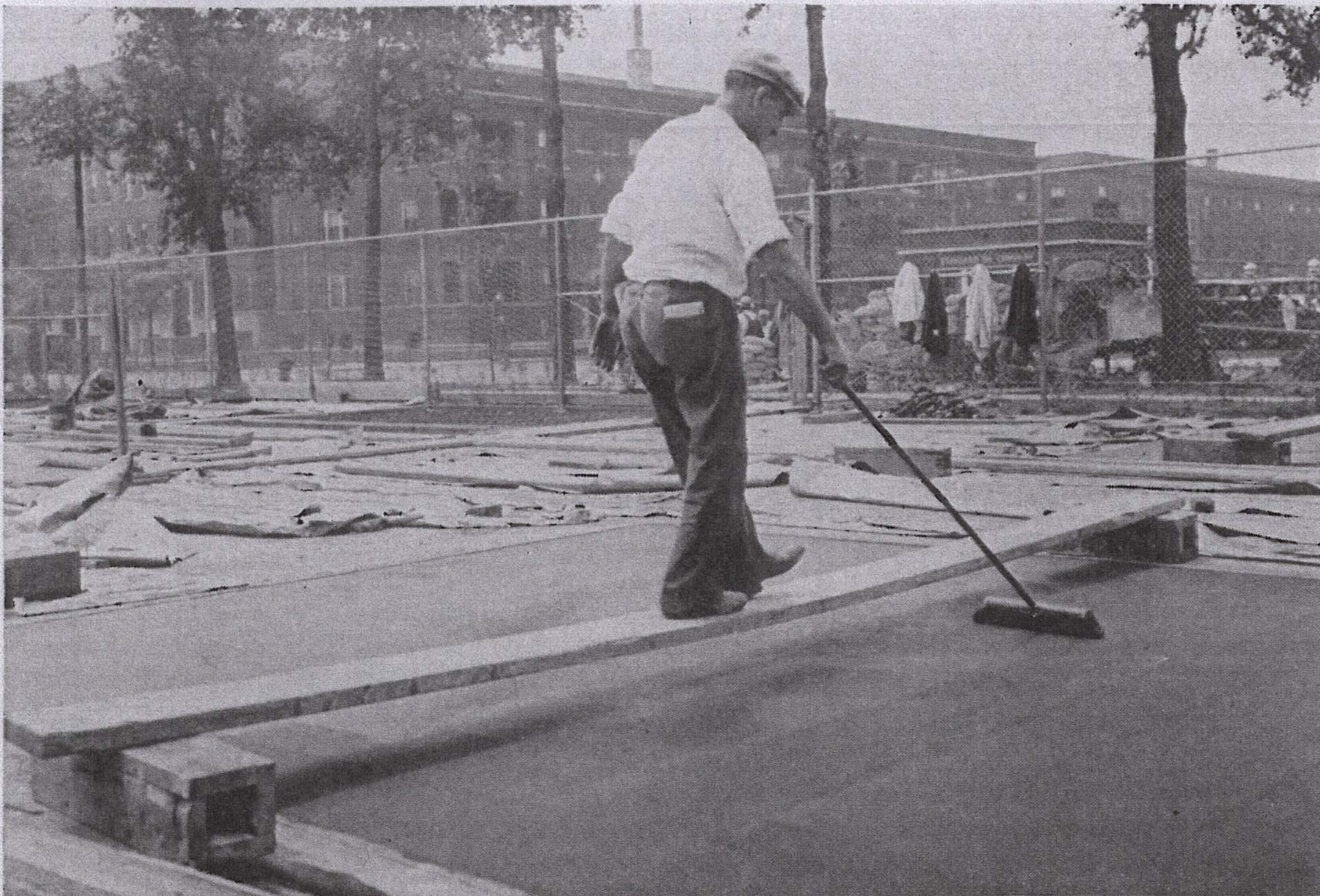
Brushing surface with floor brush in both directions to produce canvas-like finish.
