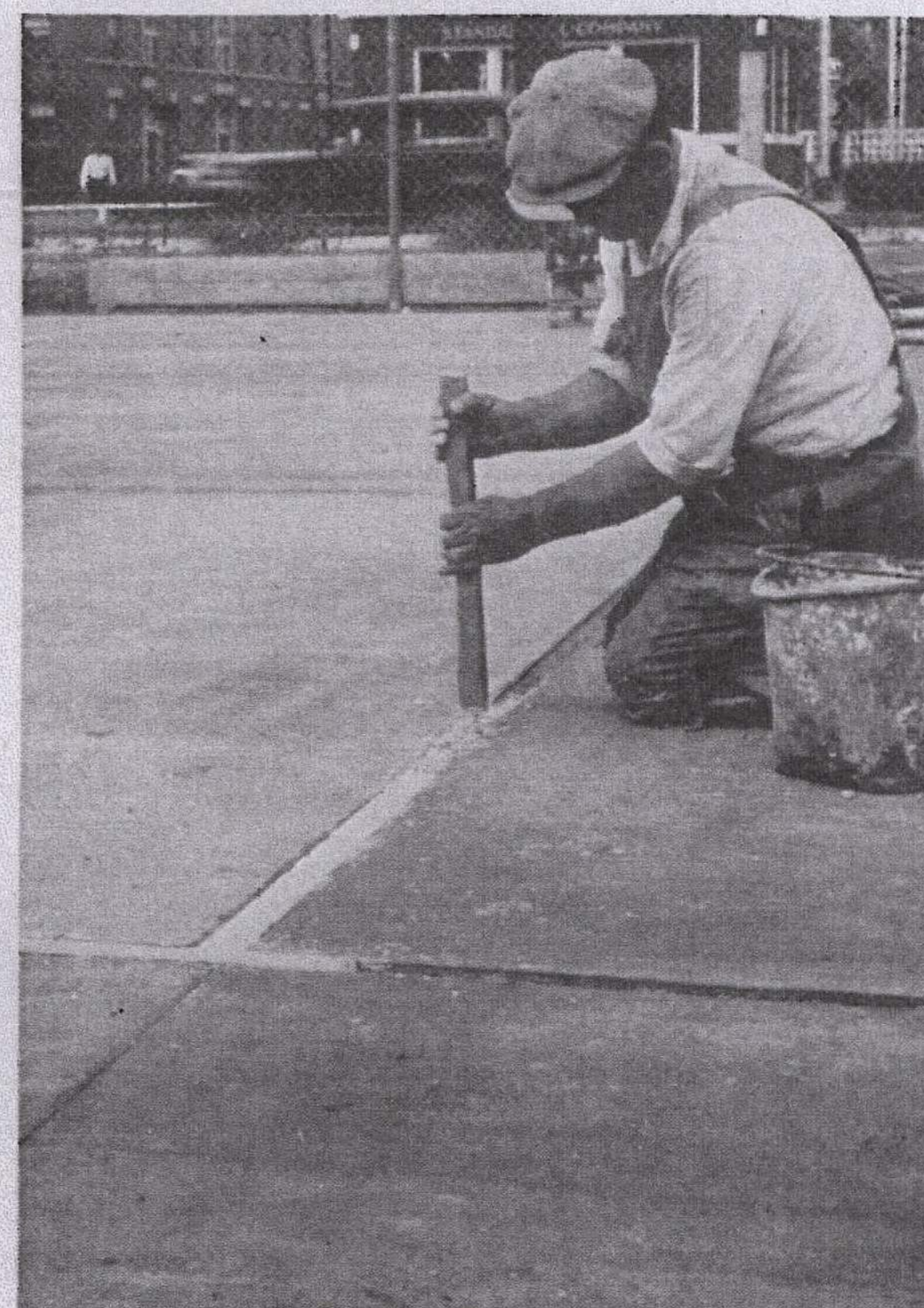
Tamping white portland cement mortar into grooves at lines.
