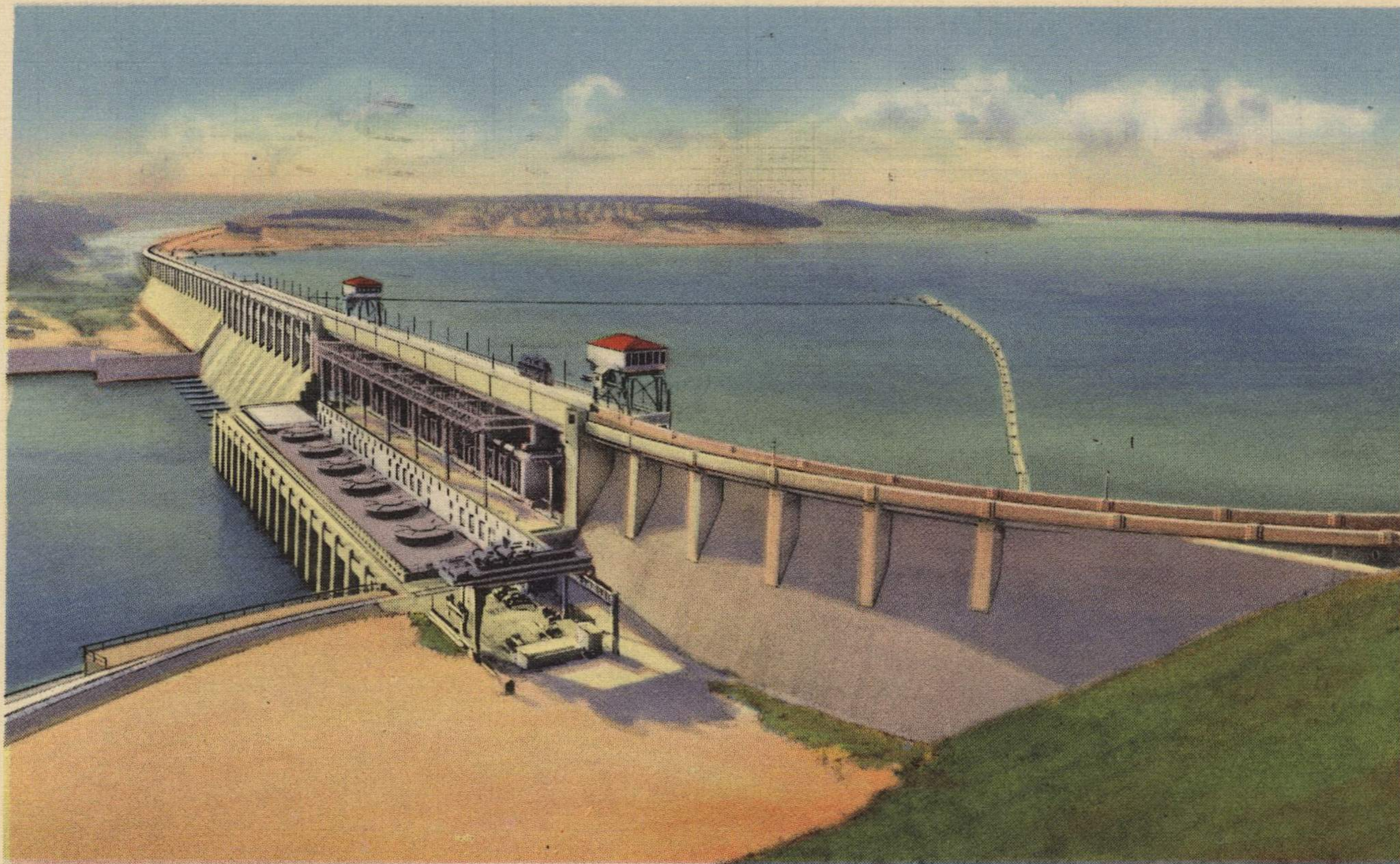
BAGNELL DAM FORMING LAKE OF THE OZARKS NEAR JEFFERSON CITY, MO.
