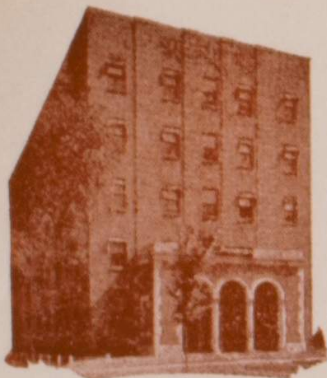
Nebraska Building Corporation, Owners
